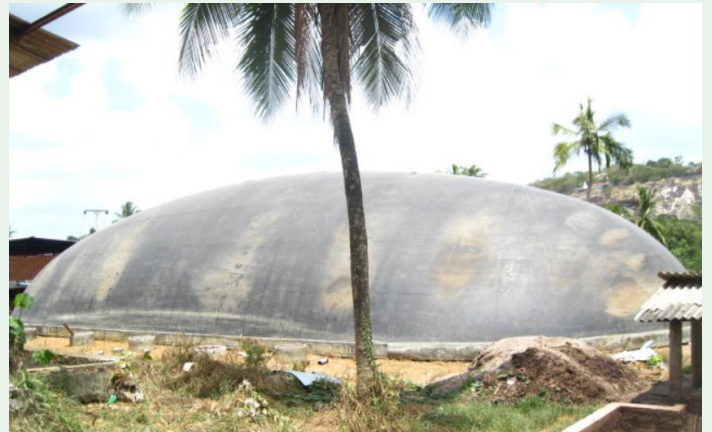
An electricity grid connected Biogas System commissioned in 2012
